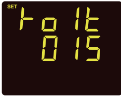
Fig 3-30 RO1 Alarm Delay Setting
